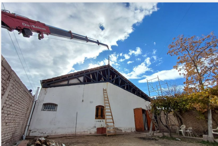
Building on the church roof
